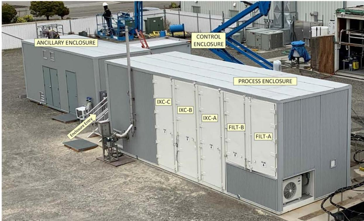
Fig. 10. FAT Enclosure Arrangement. (Final insulation/ siding not installed)
